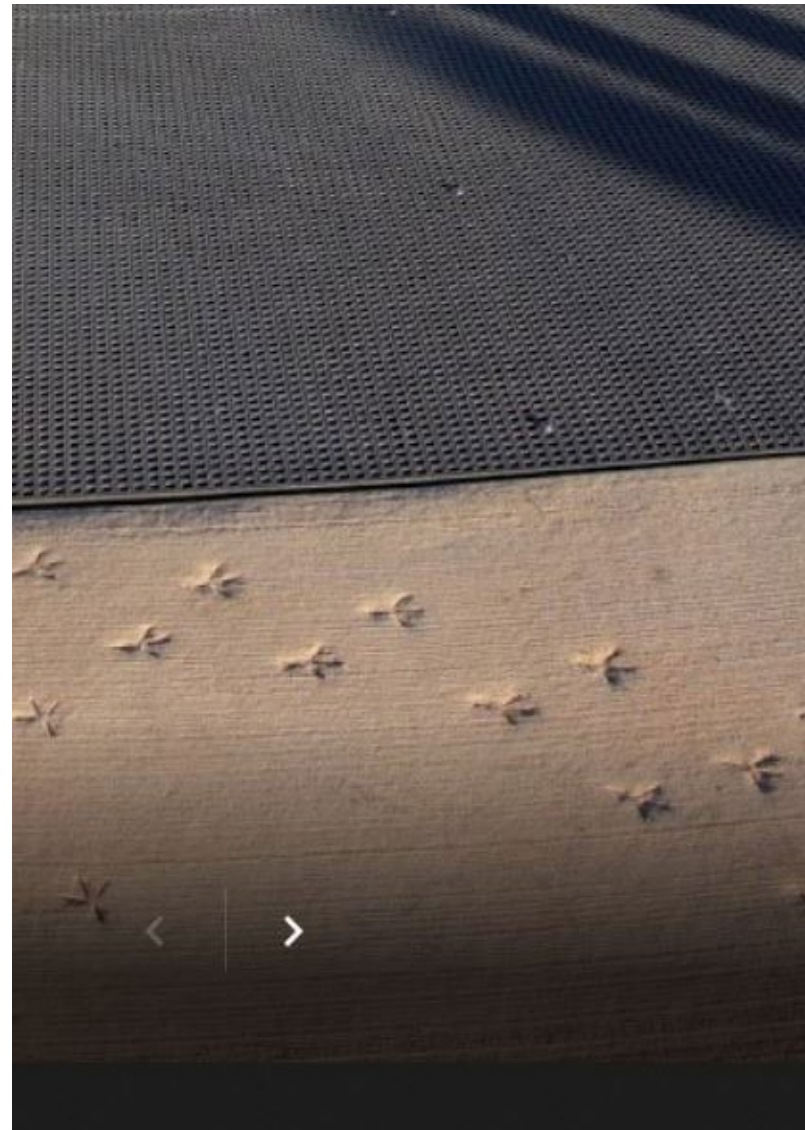
Pathway with perforated FRP deck in tree protection zone
